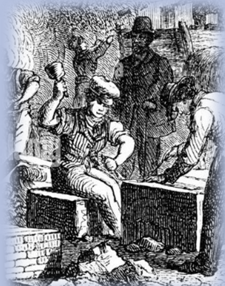
17 th century stonemason at work dressing a stone
